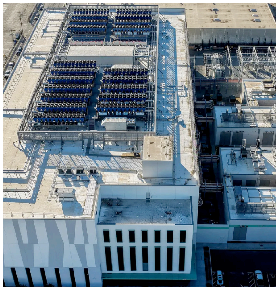
An aerial view of a 33 megawatt data center with closed-loop cooling system in Vernon on Oct. 20, 2025. A surge in demand for AI infrastructure is fueling a boom in data centers across the country. Photo by Mario Tama, Getty Images
